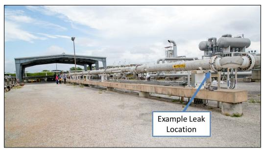
**Figure 3.1. Handheld Testing Set #1** Eight leaks were initiated at the flange pairs on a 135-ft section of straight piping.
