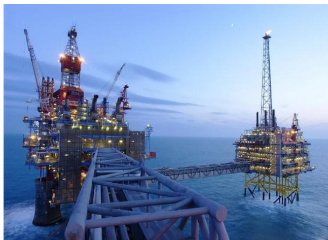
Figure 7. Sleipner A Platform. Source: Statoil
